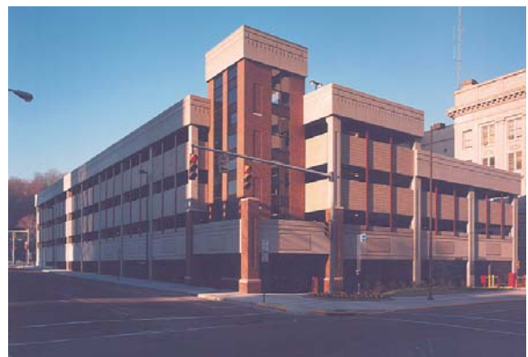
Shanklin Parking Facility
